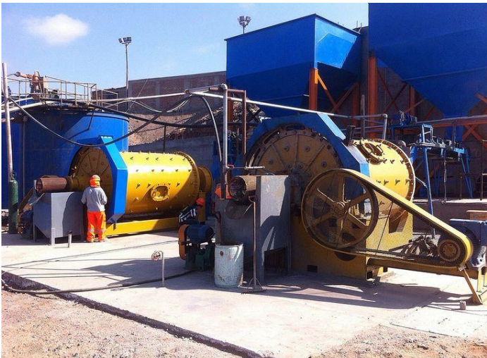
Inca One Plant ball mills and crusher circuit
